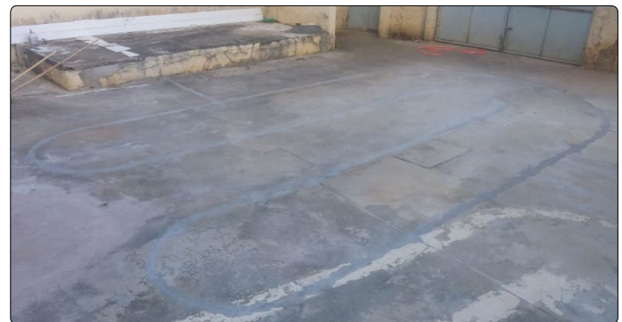
Figure 17. Wire buried in cement and covered with mortar.
